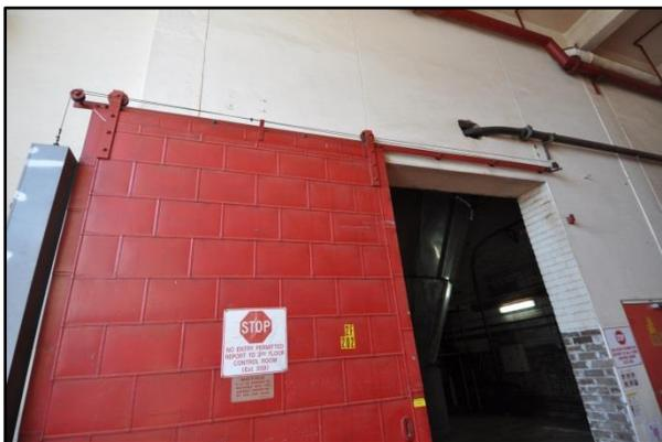
Figure 47. View of sliding steel fire escape door located on the second floor. (Source: Heritage 21, 09.03.16)
